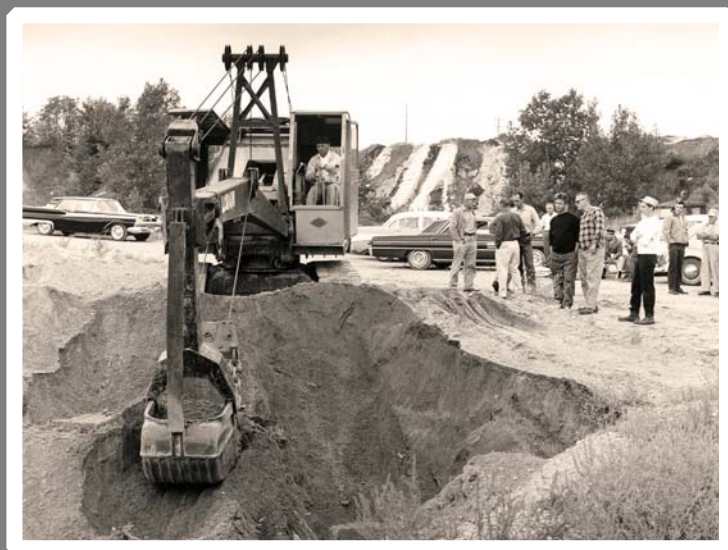
Ray Poupore running a backhoe circa 1963.
