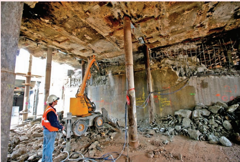
A Local 15 member operates a Broc Machine to break apart a wall on the WTC site.
