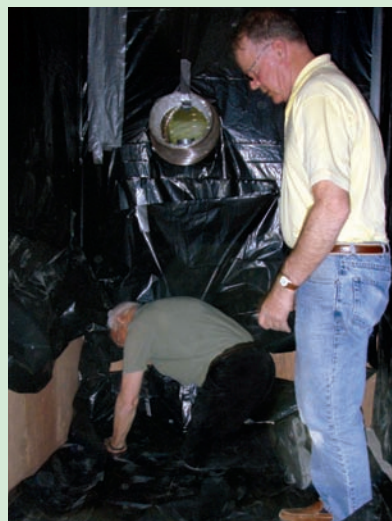
Local 4's Bill O'Neil, right, and Peter Kerrigan tape polypropylene plastic inside the asbestos training building to prepare for simulated asbestos removal from the ceiling.
