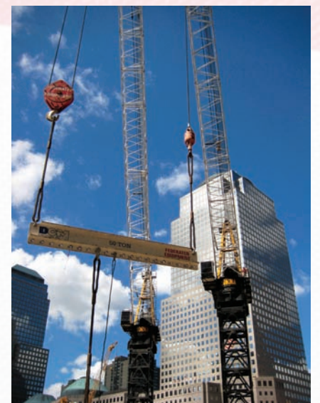
Tandem lift – Local 14 operators Ivor Hall on the crane at the left and Tim Brogan on the right set a node for the base of WTC 1/Freedom Tower.
