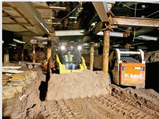
A skid steer machine, with a Local 15 operator in the seat, brings a full bucket of dirt out of the hole.
