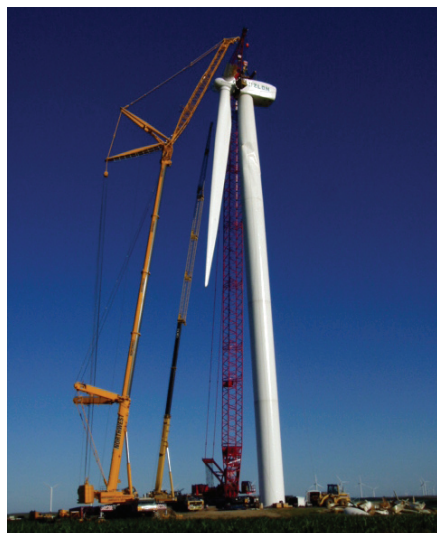
Local 49 crane operators install a wind turbine blade in southwestern Minnesota.
