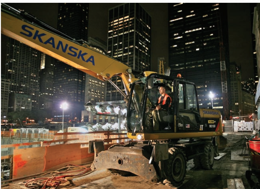
A Local 15 member operates a rubber-tired excavator at the World Trade Center site.
