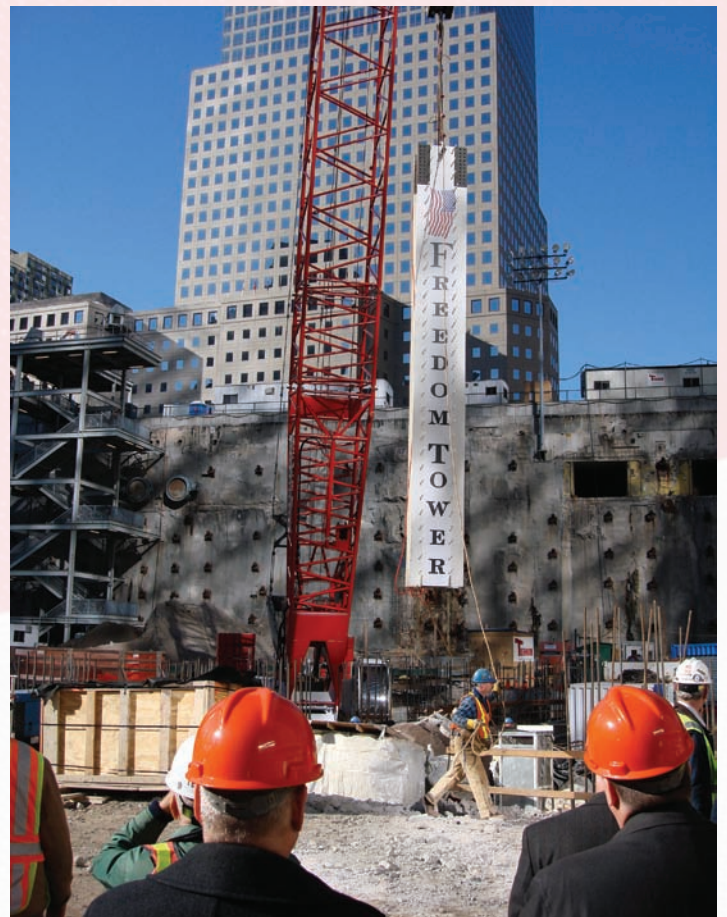
Local 14 Operator Tom Gordon on a Liebherr 1300 setting the first column at WTC 1/Freedom Tower.
