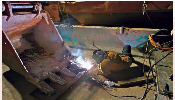
A Local 15 member welds a cutting edge onto the teeth of the bucket of an excavator.
