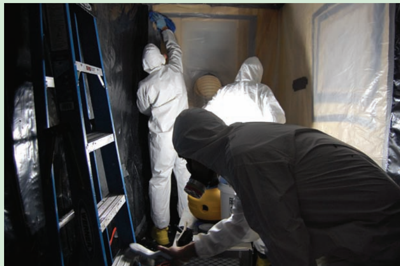
Oufitted in Level C protective gear, participants remove simulated asbestos from the interior of a unit.
