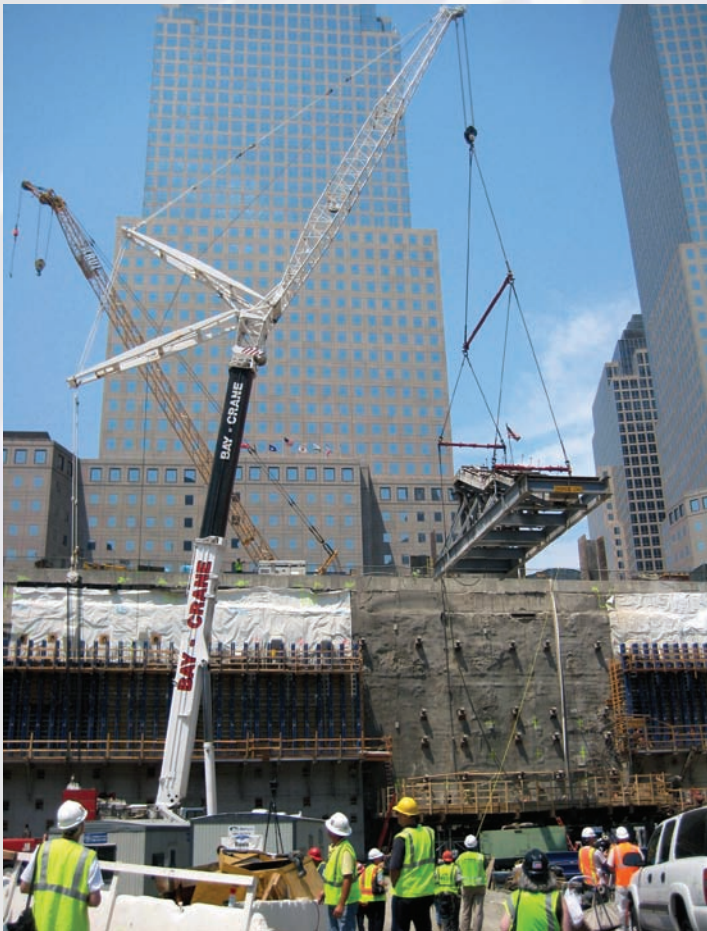
Charlie Noeth, Sr., a Local 14 member operating a Liebherr LTM1400, is setting the Survivor Staircase at the WTC Memorial. Noeth had the opportunity to have his son on the job with him. "It was an honor and a privilege to be a part of this historic event," he said. "Having been at the site in 2001 and seeing all the devastation, it felt good to be part of the rebuilding process. It was an honor to be a part of placing this important and significant piece of history in its final location. I'm proud to be a Local 14 Operating Engineer and proud to have my son as my oiler on that historic day."
