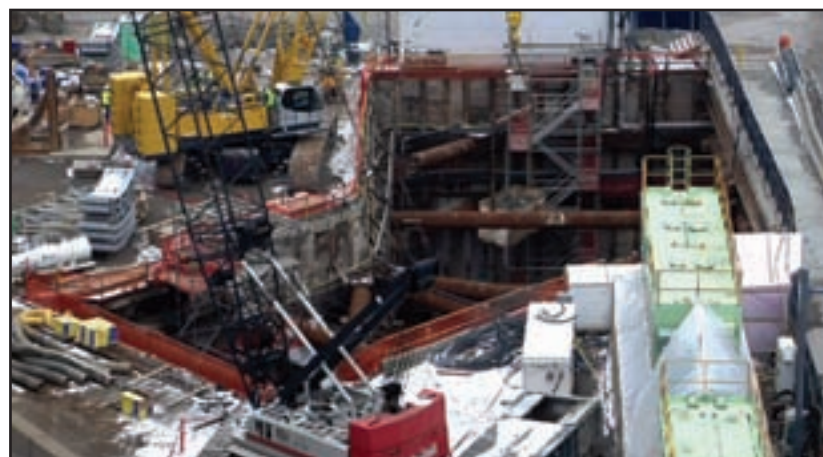
An aerial view of the project, which begins outside of PNC Park. The boring machine used cuts through the ground with crews putting four-foot segments of the tunnel behind it. Work is scheduled to end this summer.
