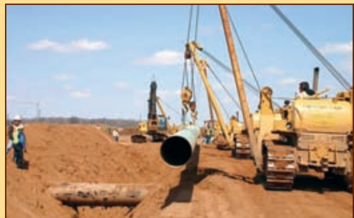
Three weeks of classes are capped off in the field with a training convoy of side-booms working in sync to lower pipe into a ditch.
